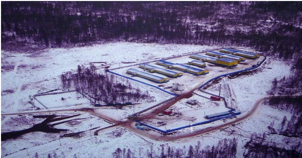
Figure 42: Installation minière d'Ozernoye (source : China Nonferrous Metal)
